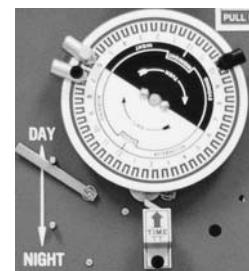
The Program Clock controls the beginning and end of the heating day.
